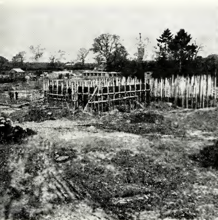
● Under construction November 1956
